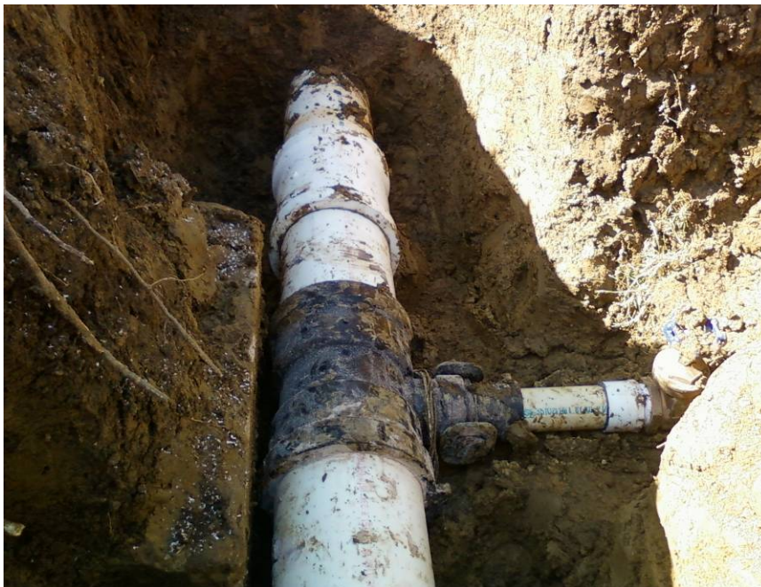
Irrigation repair of main line to #17 tee.
