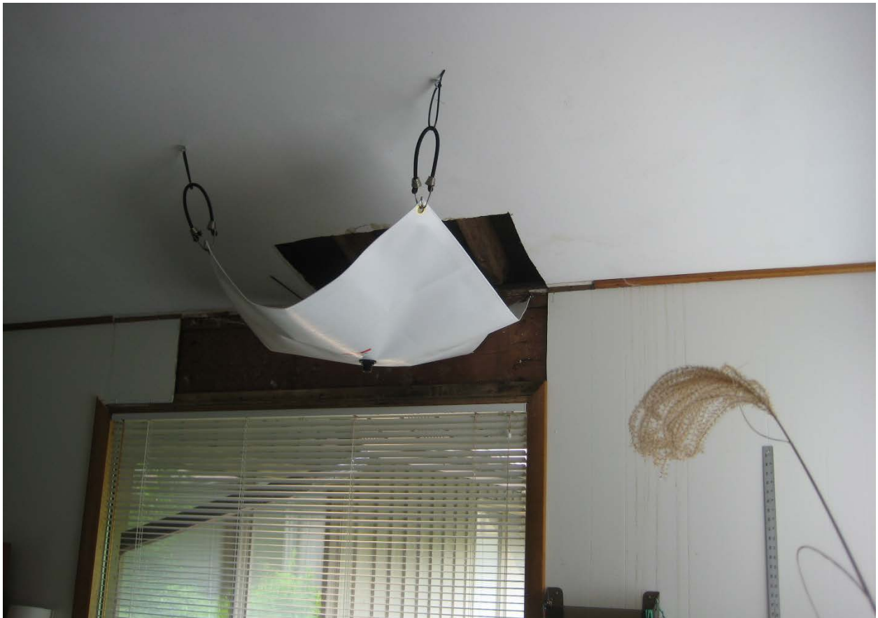
Figure 3. Damage to ceiling and wall as a result of the existing roof leak.
